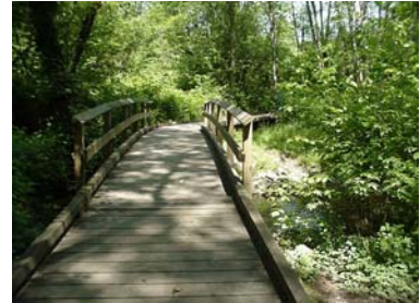
Bridge over Serpentine River
