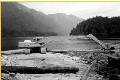
Coquitlam Reservoir – wood debris removal
