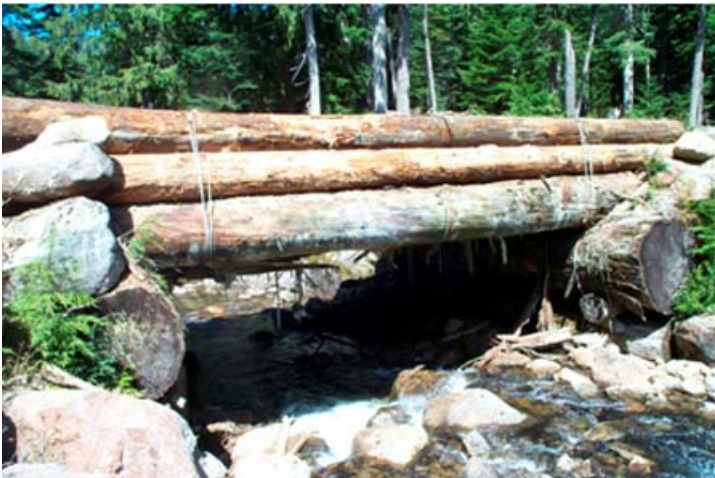
Above: Typical log bridge. Watershed staff have found a way to reuse these logs as these bridges are decommissioned, using a portable mill.
